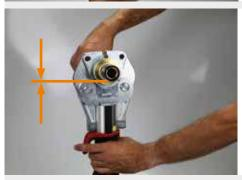
Subsequently, the pressing machine, with the third lower press jaws part, is brought into contact with the sleeve by pushing the fitting towards the machine. The fitting is then enclosed by all three parts of the press jaws.
